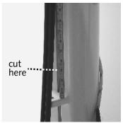
Cut the track at the mark (hacksaw included with the system hardware).
